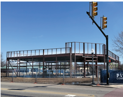
New building framing
