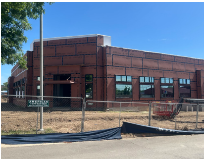
New building construction
